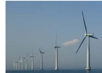
Wind turbine construction
