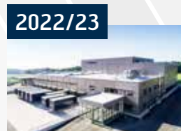
2022/23 Expansion Central Warehouse
